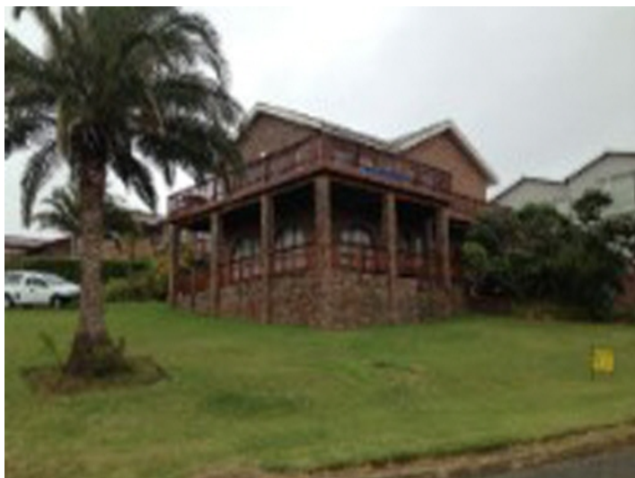
General view of the property
